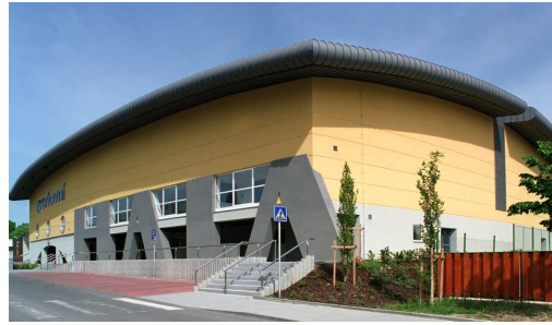
Outside view of the Sport Centre
